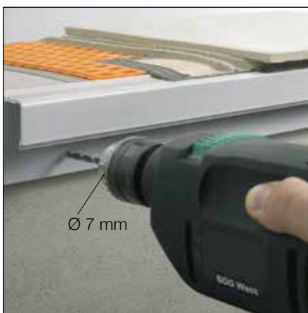
Subsequent installation of the Schlüter®-BARIN gutter system to the edging profile
