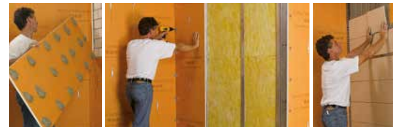
Substrate, structural panel, bonded waterproofing
