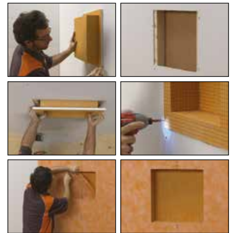
Installation in drywall
